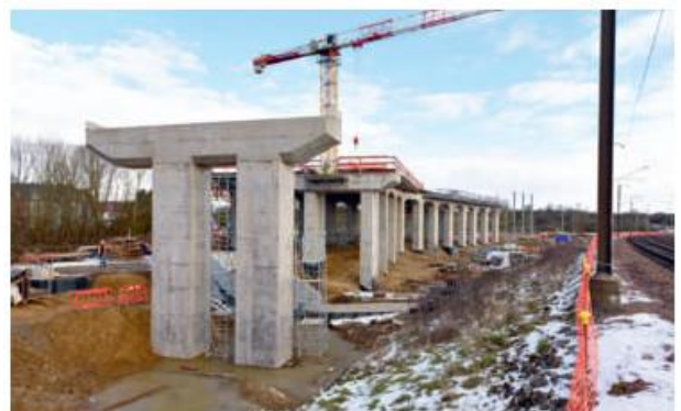
Overpass north of Bettembourg for the new line to Luxembourg (CFL)
