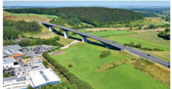
N11 bypass, Junglinster, opening 2015 (P&Ch)
