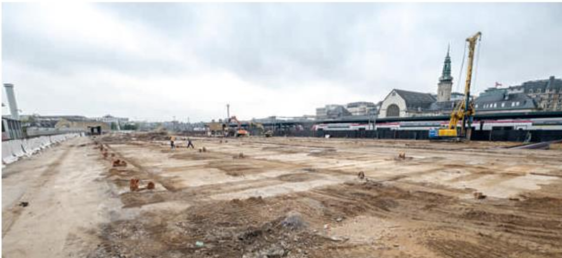
Expansion of the Central Station (CFL)
